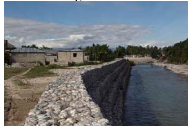
Courtesy of UNDP : gabion walls
