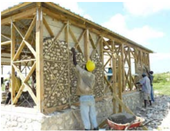
Courtesy of UNDP Filing of walls with recycled debris
