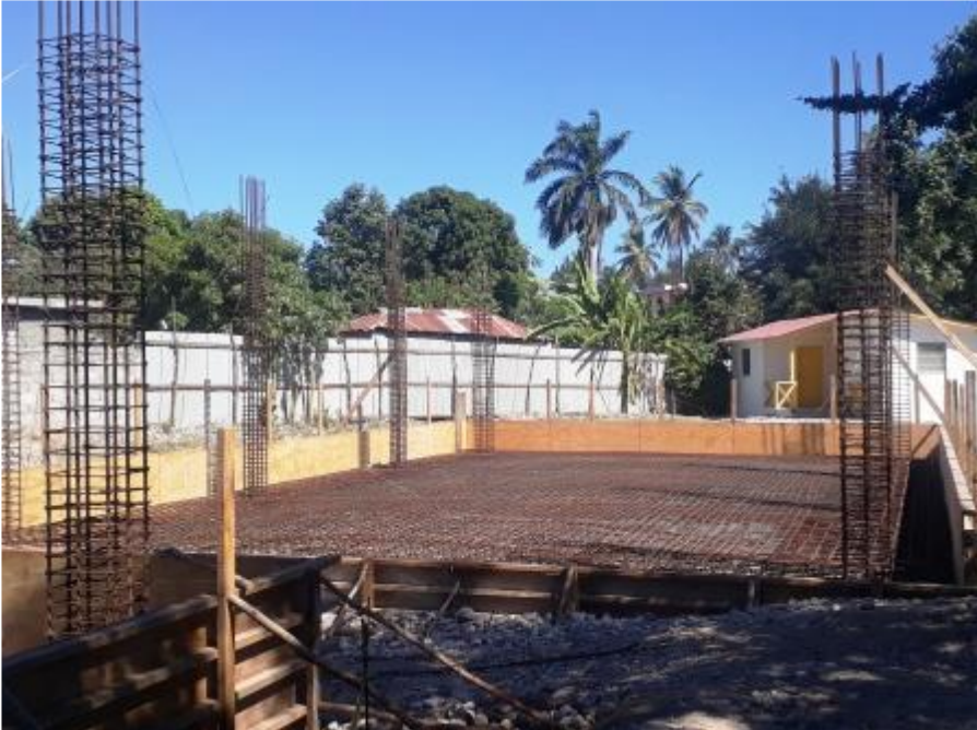
Finished reinforcement awaiting the pouring of concrete
