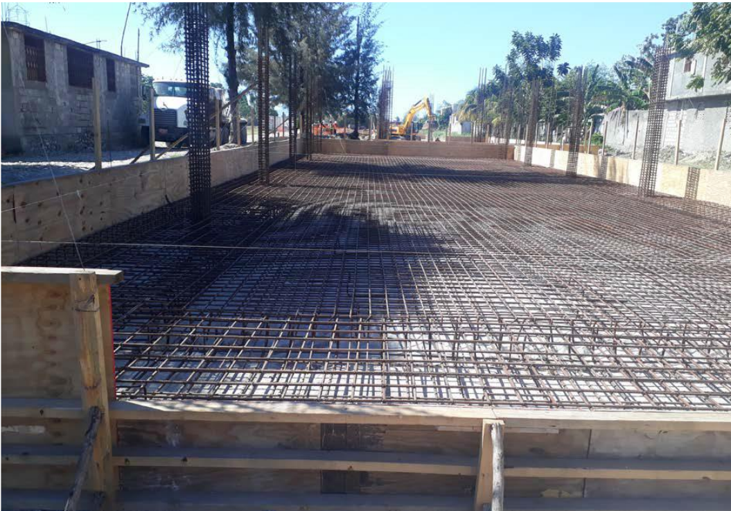
Finished reinforcement awaiting the pouring of concrete
