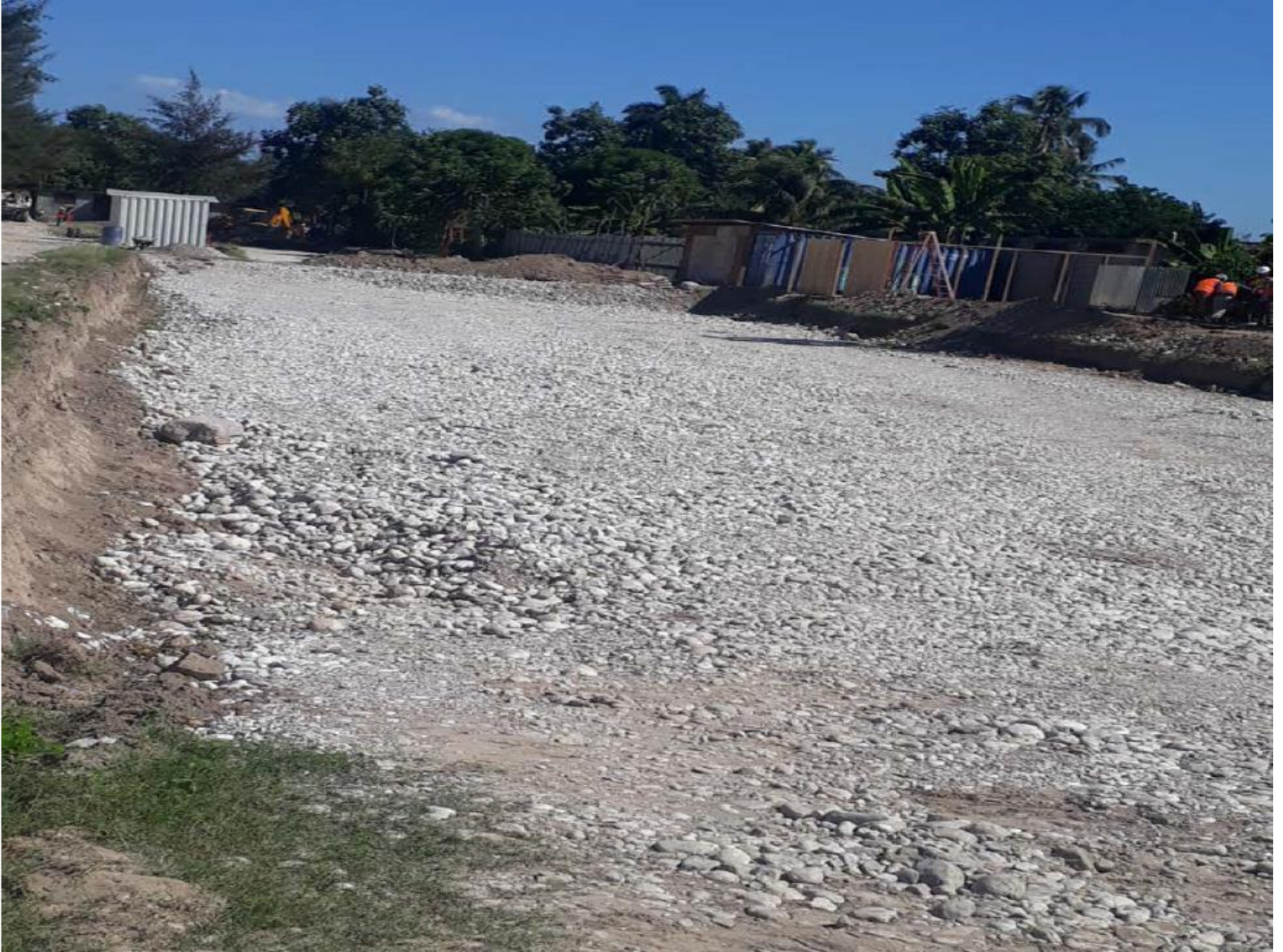
Second layer of backfill in classrooms awaiting compaction test by the building laboratory (LNBTP)
