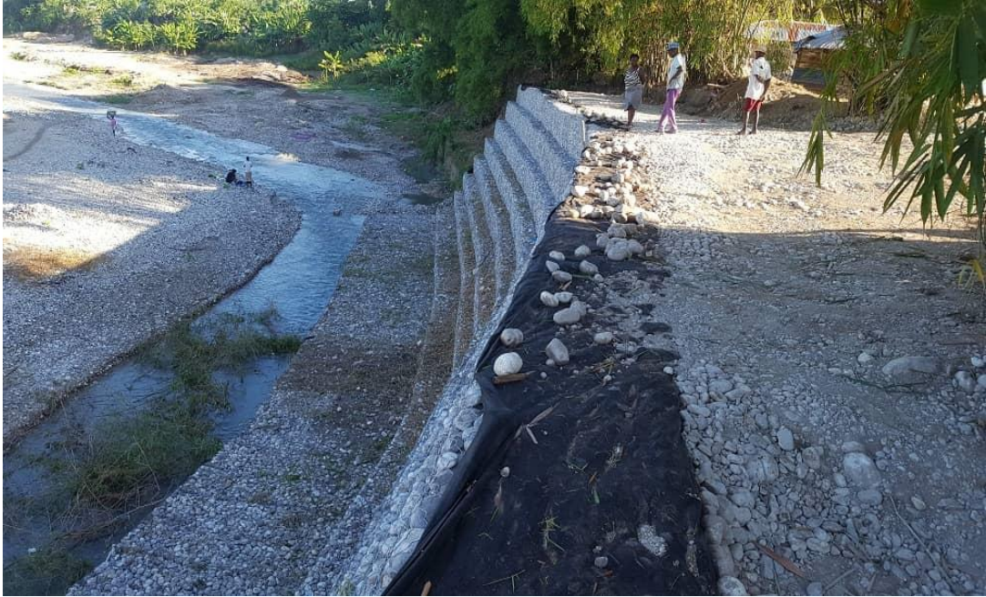
Gabion protective wall in the river
