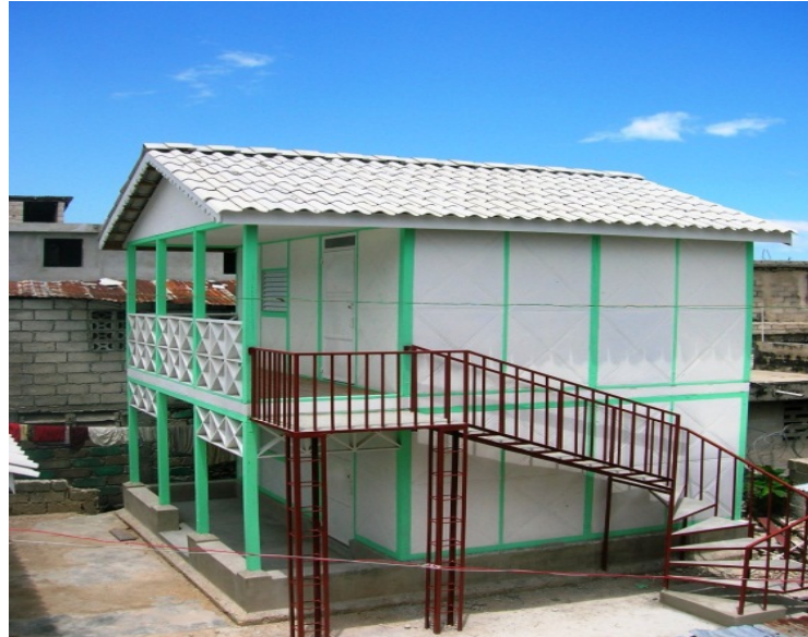
House built out of recycled debris. Carrefour-Feuilles, Port au Prince – Courtesy of UN
